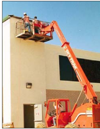
SAFETY WORK PLATFORM
